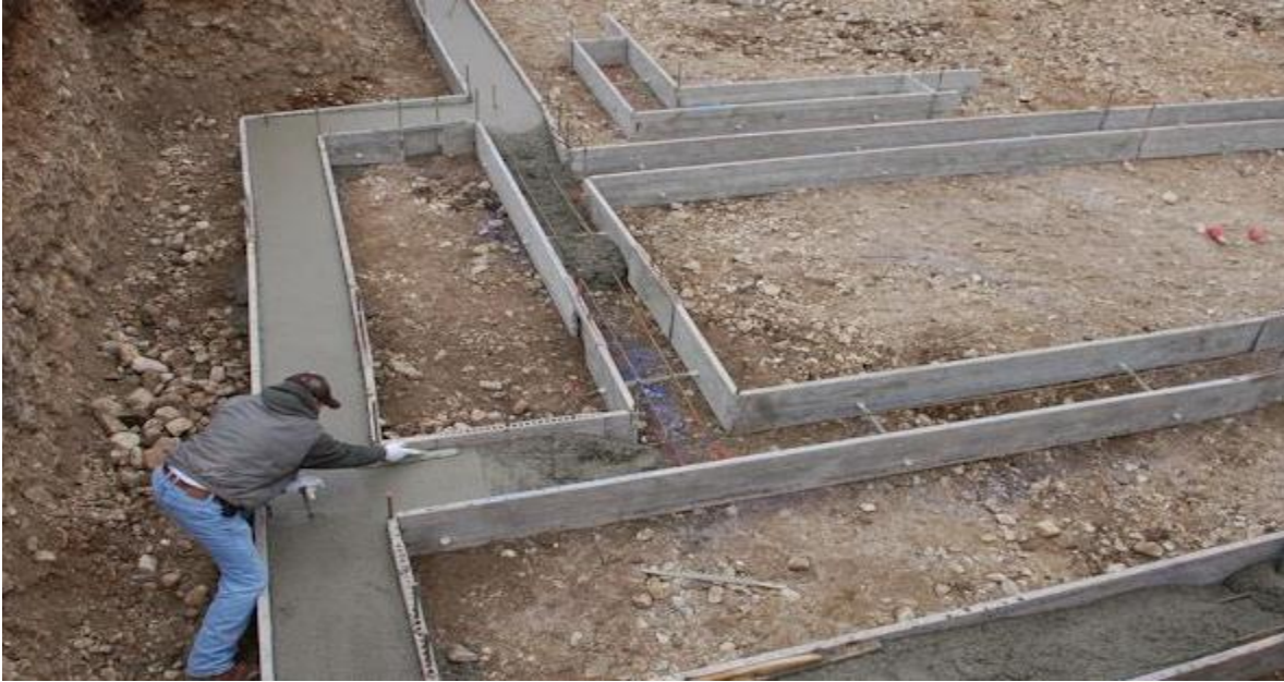
Figure 9 Wall Footing or Strip Footing Image
