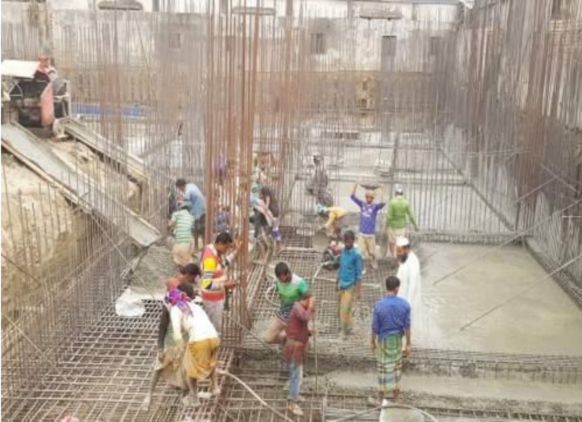
Figure 12 Raft or Mat Foundation Image
