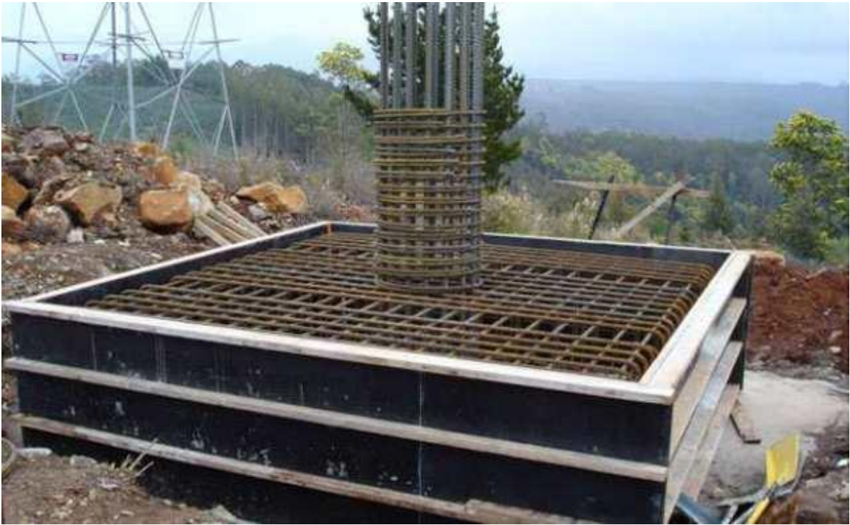
Figure 8 Grillage Foundation
