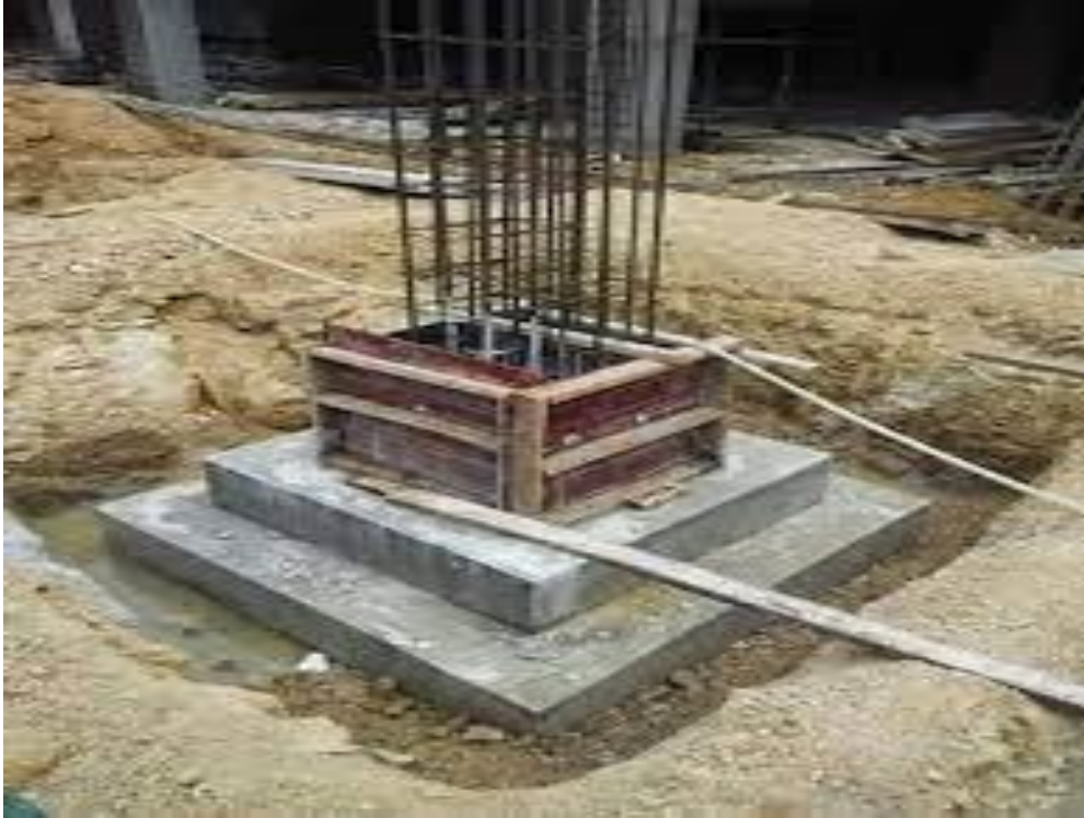
Figure 4 Stepped Footing for a Column
