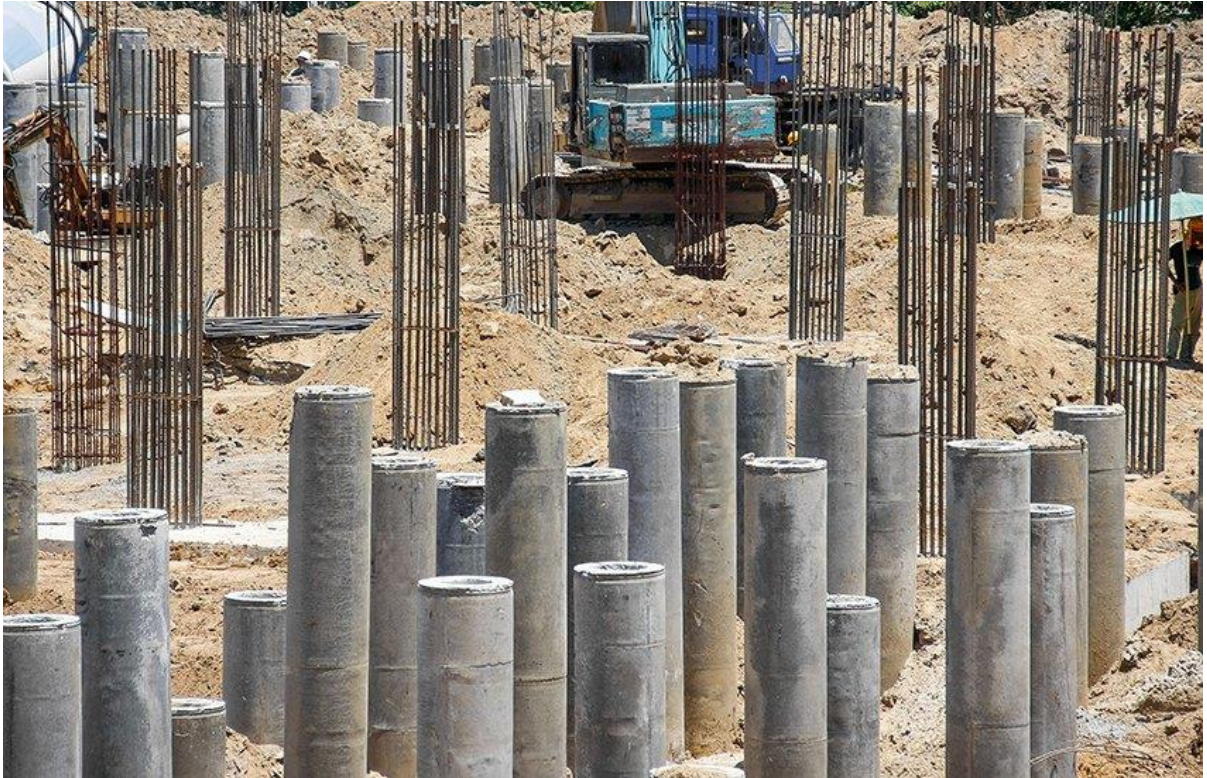
Figure 23 Concrete Pile Image
