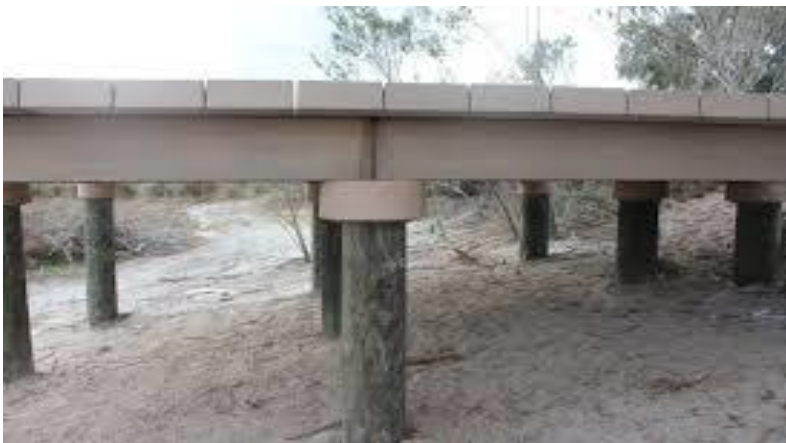
Figure 22 Timber Pile Image
