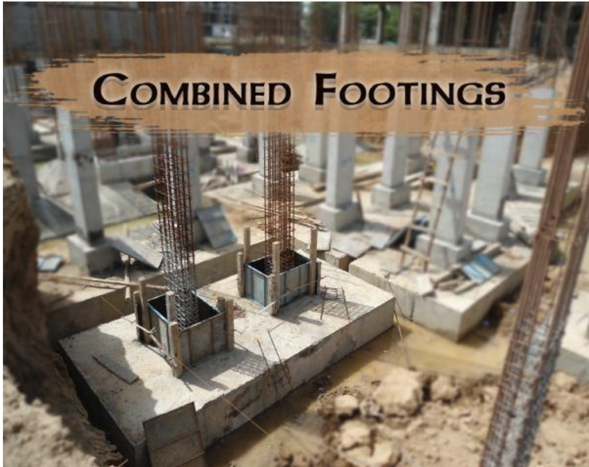
Figure 10 Combined Footing Image
