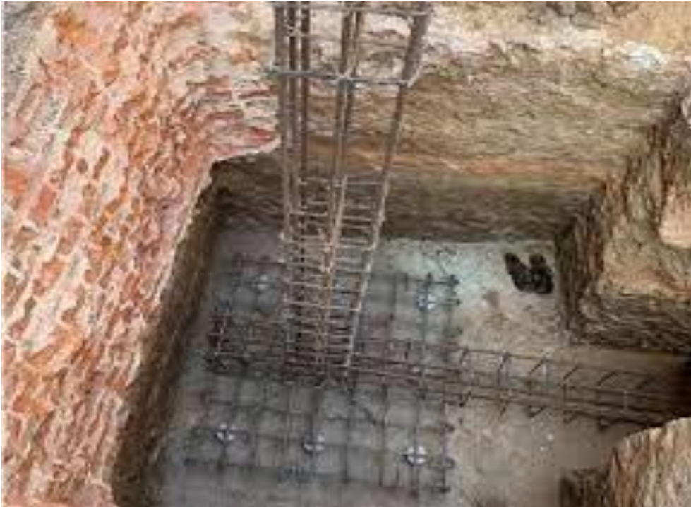
Figure 11 Cantilever or Strap Footing Image
