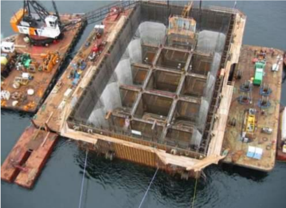
Figure 27 Caisson Foundation Image
