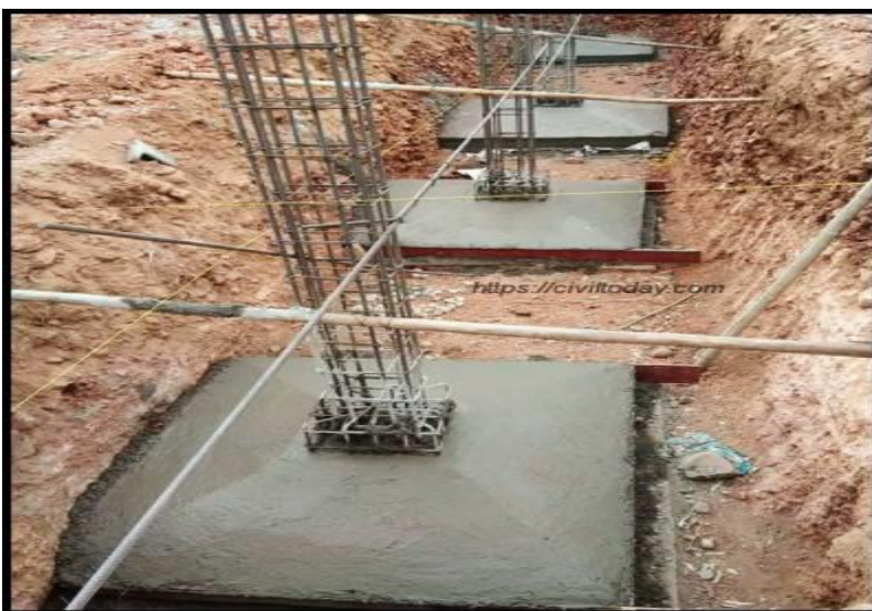
Figure 2 Isolated Shallow Foundation Image
