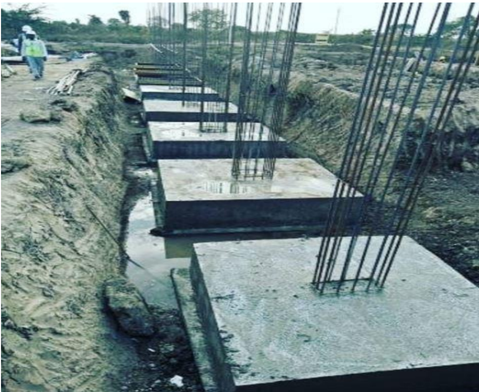
Figure 3 Single Pad Footing
