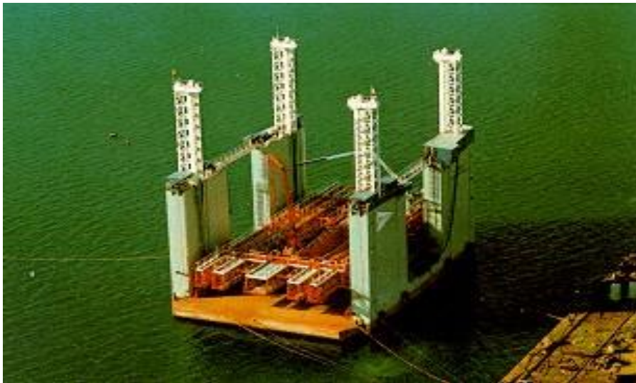
Figure 29 Floating Caisson Image
