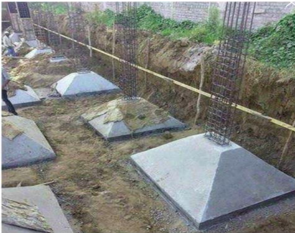
Figure 5 Sloped Footing for a Column
