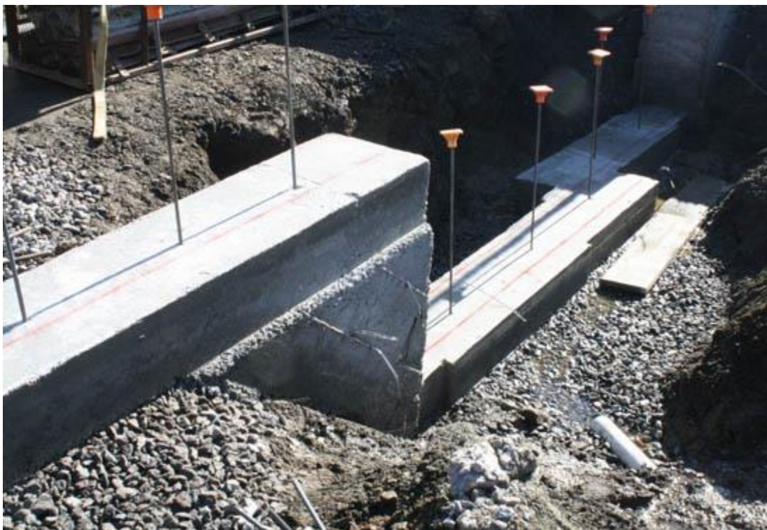
Figure 6 Wall Footing without a Step
